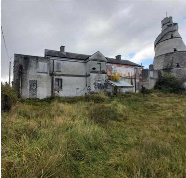
Figure 21 - View of the rear of the barn
