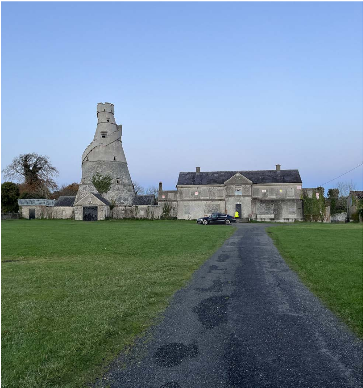
Figure 34 - The Wonderful Barn and Barnhall House
