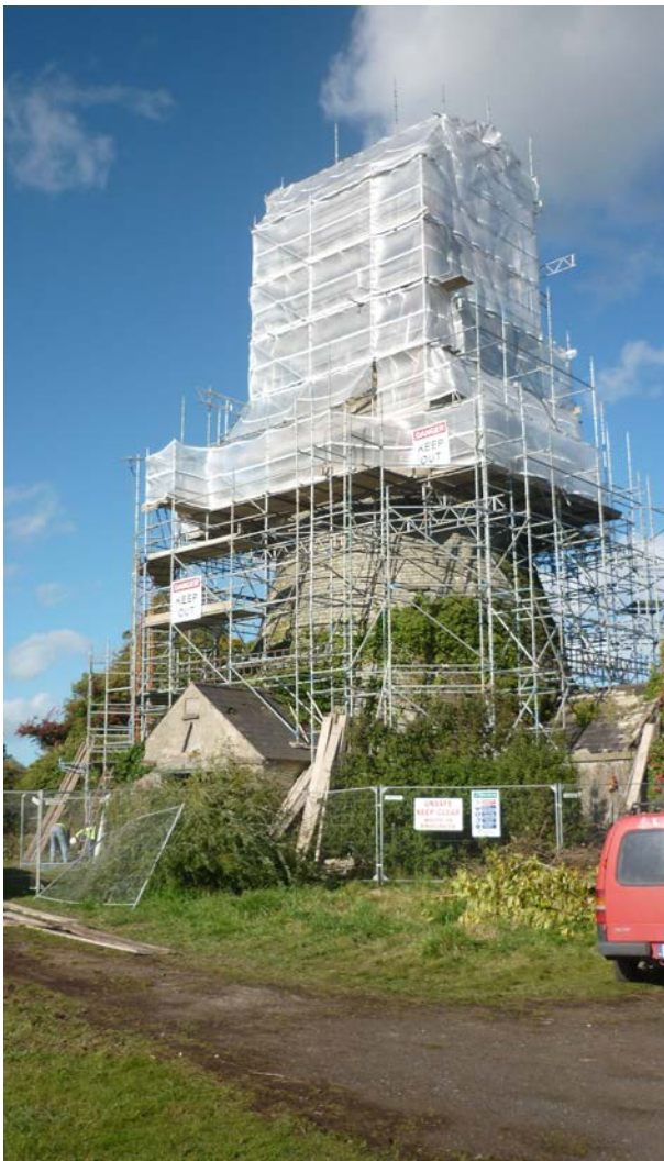
Figure 35 - Repair works carried out to the Barn in 2005
