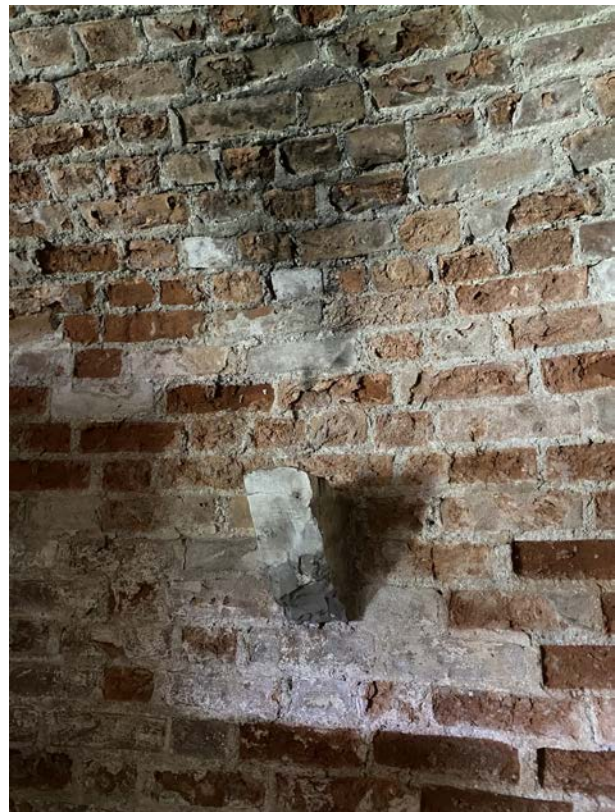
Figure 36 - Internal brickwork in the ground floor of the barn
