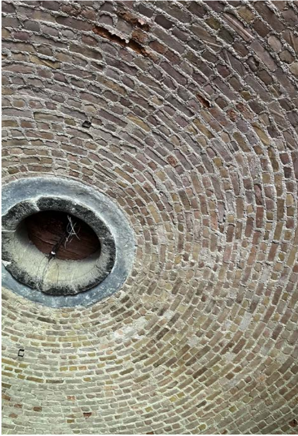
Figure 15 - The vaulted brick ceiling of the ground floor with central opening for grain
