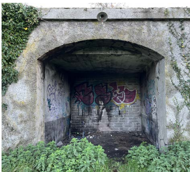
Figure 27 - Archway in the north-south running stable range, infilled with blockwork
