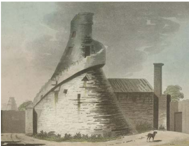
Figure 32 - Halls Barn in Churchtown (1795)
